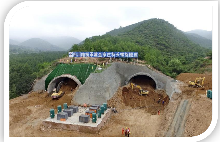
Yanqing – Chongli Expressway under construction
